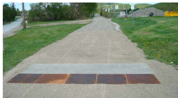
Newly installed truncated dome
