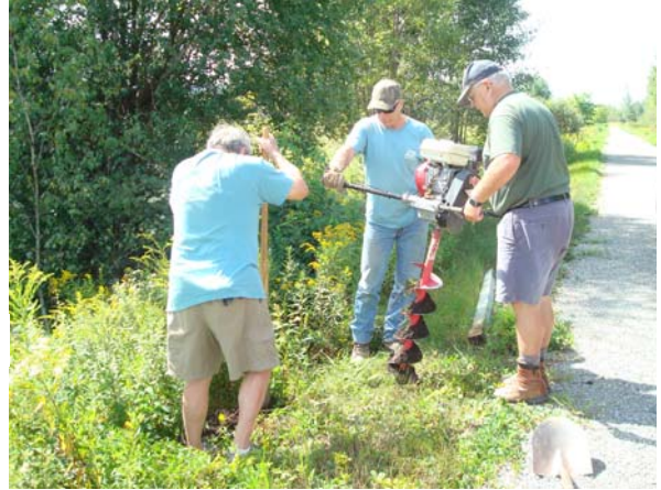
A very heavy auger was used to drill the holes for the mile marker posts
