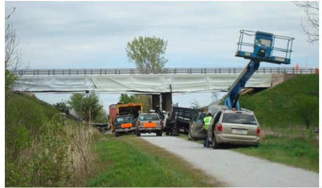
Bridge painting equipment on the MVRT
