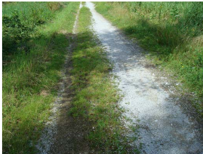
After resurfacing, the Trail will once again be 10' wide.
